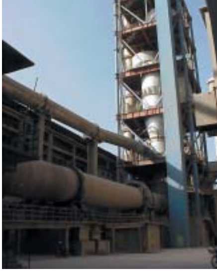
Figure 2: new kiln and preheater-precalsiner tower
